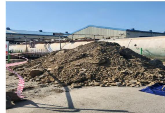
Separate storage of excavated soil surrounding the condensate water storage tank
